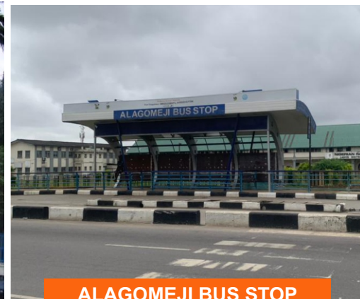
ALAGOMEJI BUS STOP
